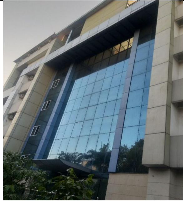
C6 - Glass building
